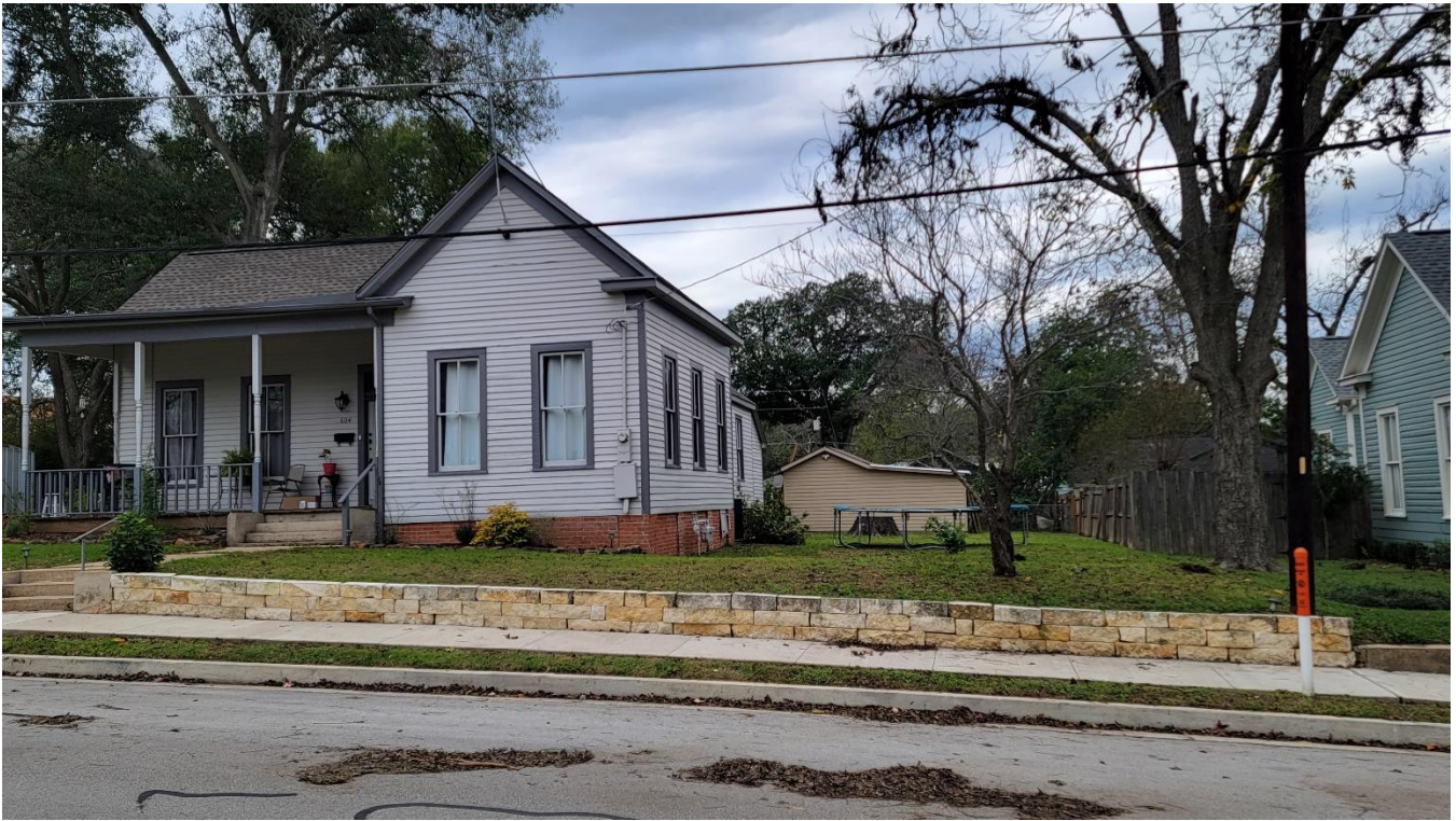
North side of the subject property- Can see back dividing chain link fence.
